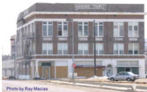
North side of the building
