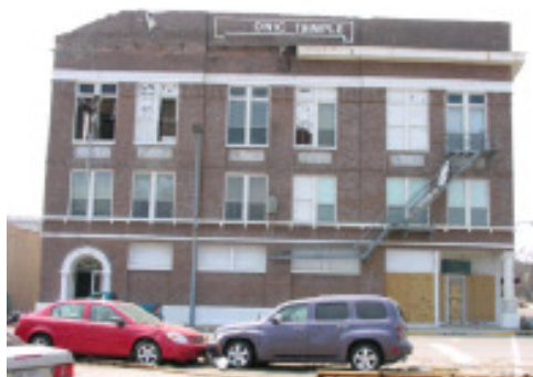
East Side of the building
